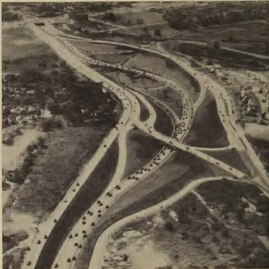
Ramps may be of different forms, but the two general classes are inner loops and direct connections.
